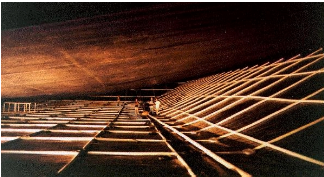
Figure 4.3 - View under the cover of the pond. The PVC frame to which the positively buoyant PMTs are mounted can be seen.
