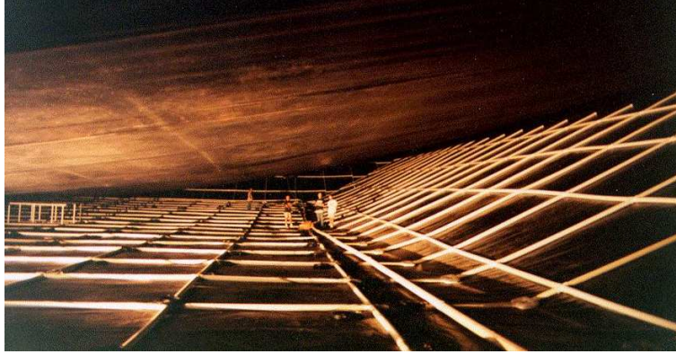
Figure 2.1: Inside the Milagro pond, before any PMT installation. The pond is about the size of a gridiron football field. The grid positions correspond to eventual PMT positions.
