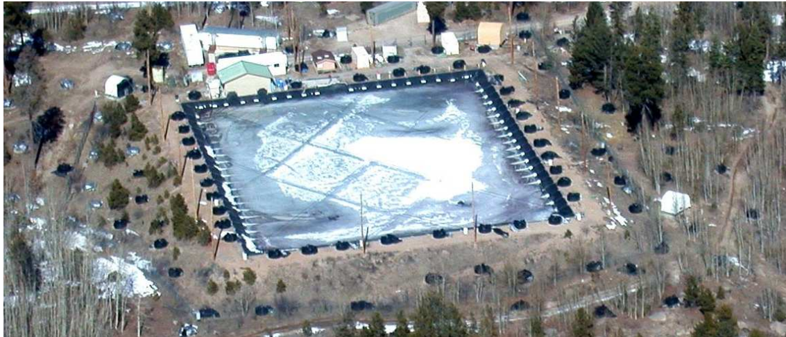
Figure 3.1: The Milagro site in the Jemez Mountains of New Mexico. The central, covered pond is surrounded black outrigger tanks. Some snow is visible on the cover.
